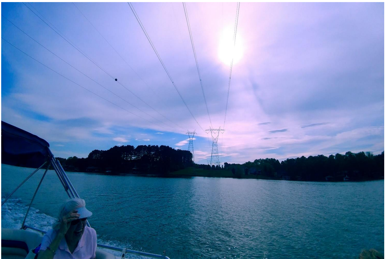
Figure 5: TVA Powerline Crossing at Mile 6 of Tellico Reservoir
